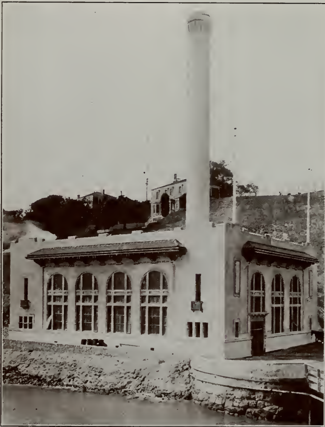
FORT MASON PUMPING PLANT
